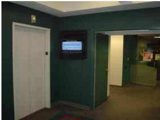
Elevator Bay Installation
