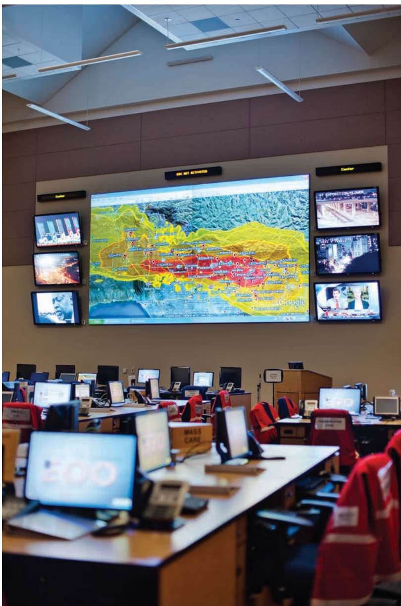
Spectrum began a one-year programmatic design for the EOC in 2003 and returned to design the systems in 2006, oversee the AV contractor, and do commissioning and testing over a continuous four-year period. Photo by Brad Howell
