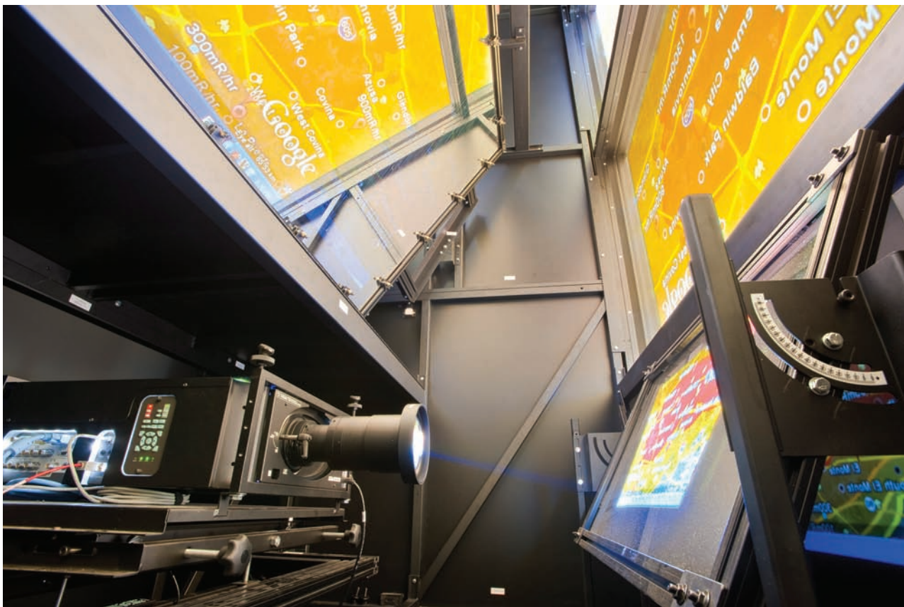
Housed in a unique seismic-rated display structure by RP Visuals, four 10,000-lumen Digital Projection International Titan 1080p-700 3-chip projectors do the heavy lifting for the main display wall. Photo by Brad Howell
